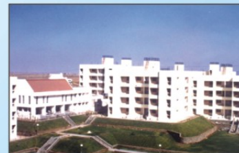
PUNE (Ph-I) - 159 DUs Completion Year : 2003
