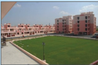
LUCKNOW - 130 DUs Completion Year : 2008
